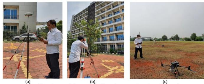
Field Work Image : (a) GNSS CORS, (b) Total Station Reflectorless, (c) UAV Lidar
